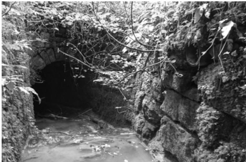
covering the whole floor. It is big enough for a fully grown man to walk upright all the way through, and could be 250 to 300 feet long. The entrance with its winged entrance walls, some ten feet tall has a stone and debris trap at the tunnel's opening. The tunnel (pictured) could be as much as 50 feet below the main road.
