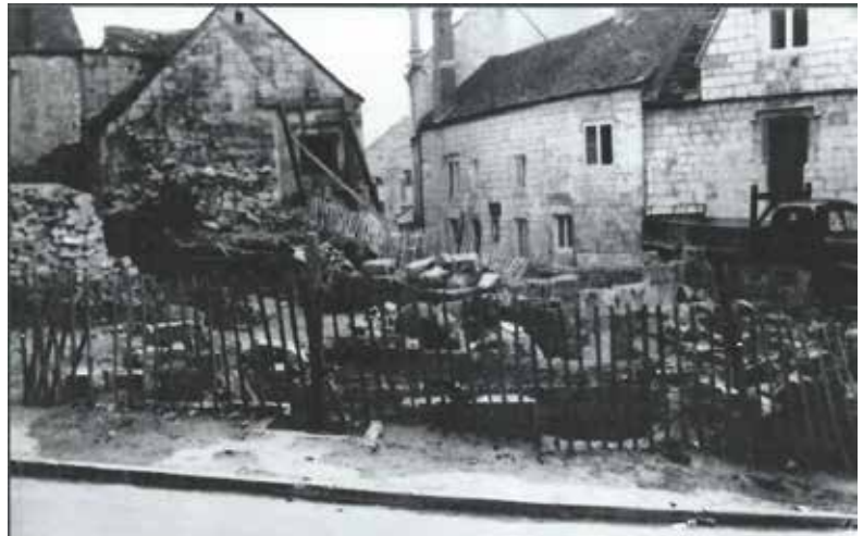
Looking across the bomb site from Friday Street to the Royal Oak
