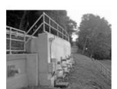
Fig. 2 West End of new retaining wall with tension
