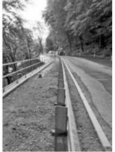
Fig. 1 Safety Barrier in place between carriageway and retaining wall
